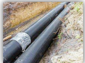
Pipeline Leak Detection System
